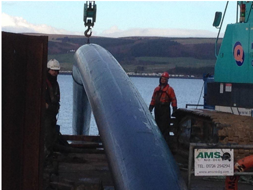
Pipeline positioned on the sea barge during installation
