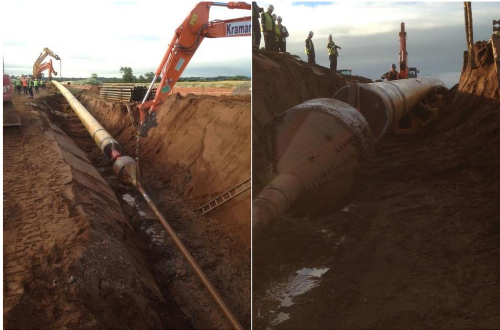
*36 inch steel pipe being pulled into position ready for installation*
