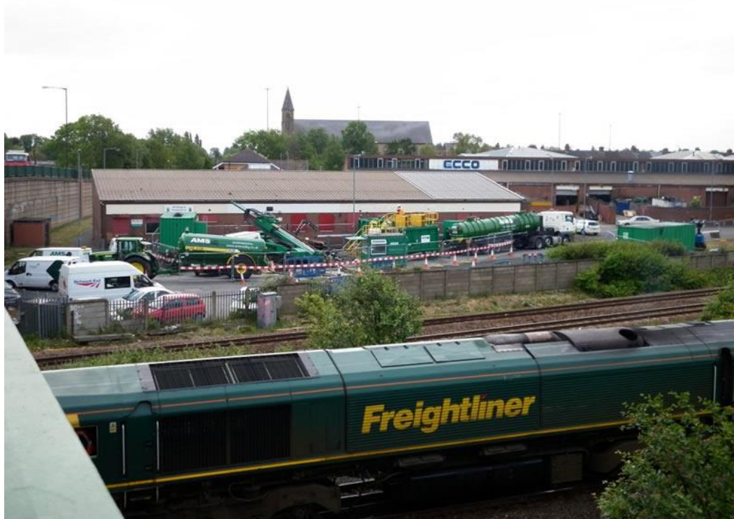
View showing the drill line beneath the live railway lines
