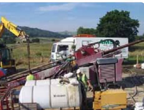
The contract was commissioned by Murphy Pipelines and consisted of a single drill of 8" steel for 340m under the River Severn and two of its tributaries.
